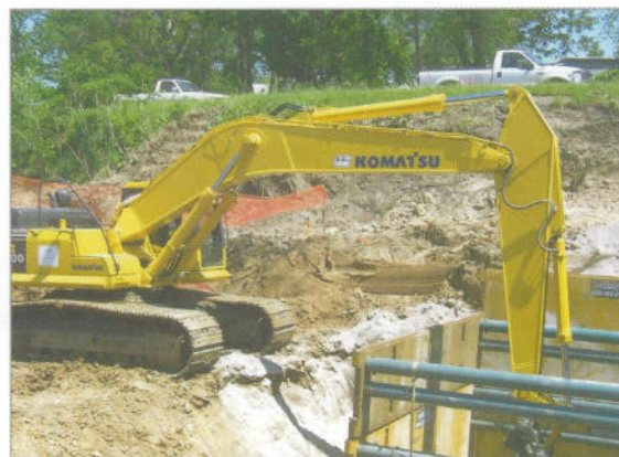
A Fahey track hoe gets down to business at Penn Valley Park.
